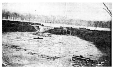
The quarry dike breaks. Note floating tank cars.
