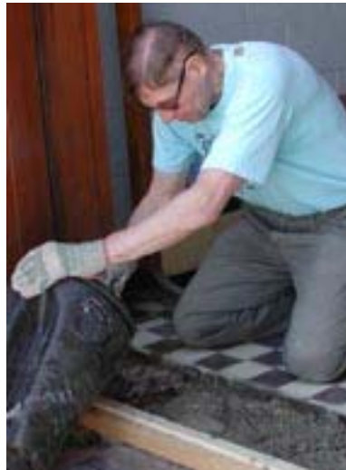
Dave Cooney putting in a new cement threshold.
