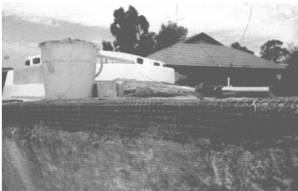
..the same joint ready for re-plastering
