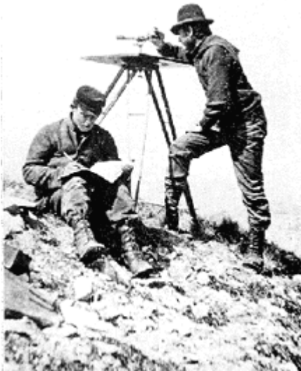
Planetable surveying by turn-of-the-century USGS topographers
